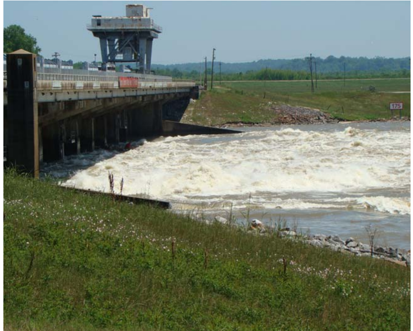
Water flowing into the Atchafalaya River at Old River Control Structure
