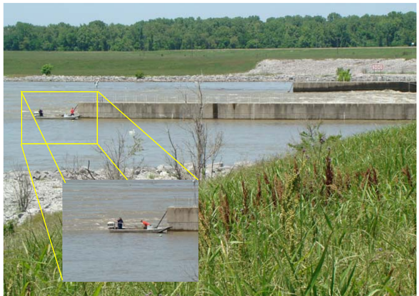
Water flowing into the Atchafalaya River at from the Auxiliary Control Structure of the Old River Project. Note the fisherman at the end of the structure. The fish must be biting good to get them out there!
