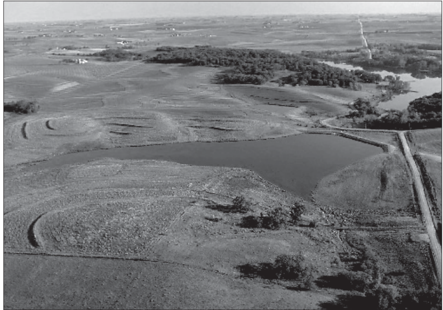
Figure 34-31. A small dam, terraces, buffer strips, and grass plantings are designed to improve the quality of water entering a lake.
