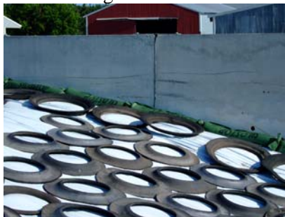
Figure 2. Plastic drain pipe used to cover the top of the wall to prevent side wall plastic from being torn or punctured.
