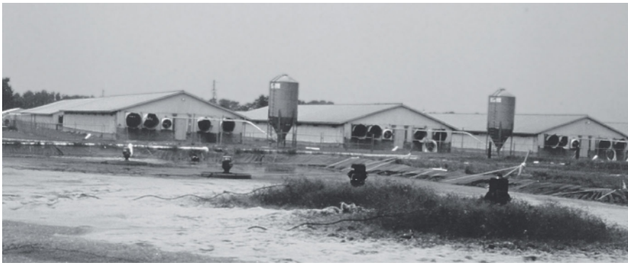
Figure 43-8. Aerated lagoons treating flushed swine manure.
