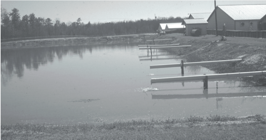
Figure 43-10. Partial view of an anaerobic lagoon treating swine manure.
