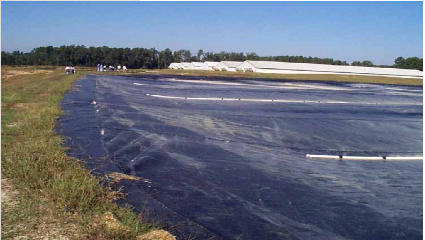
Figure 3. Negative air pressure and floating manure storage covers require a system to collect and remove rainwater and snowmelt. (Source: Ron Sheffield, Louisiana State University)
