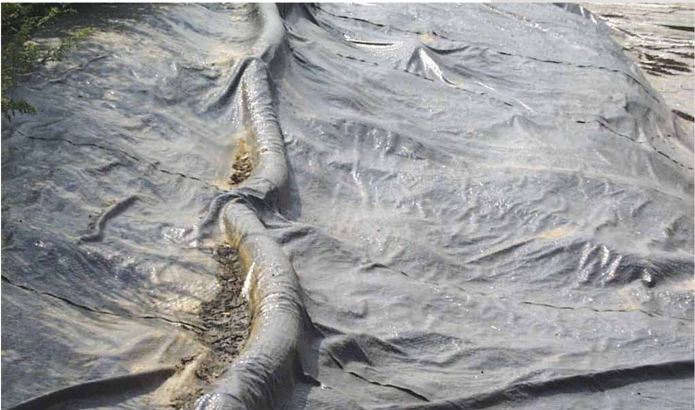
Figure 2. Negative air pressure covers are held in place by a vacuum created by fans that pull air out from under the cover.
