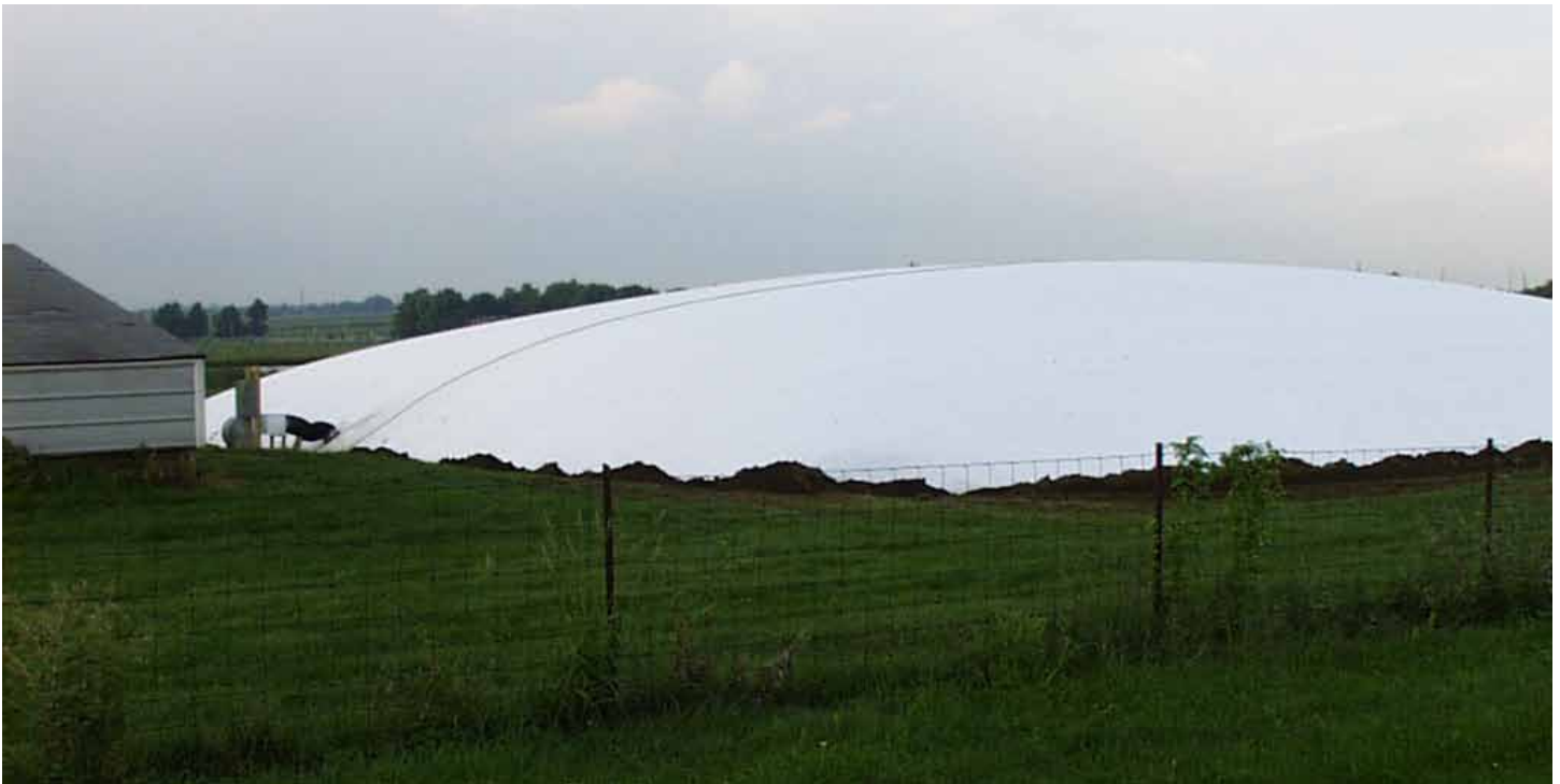
Figure 1. Positive air pressure covers are filled with air from a blower. (Source: Ted Funk, University of Illinois)
