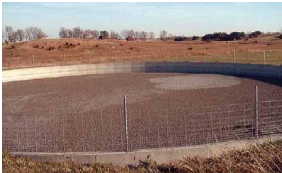
Figure 3. A permeable manure storage cover made of lightweight expanded clay aggregate (LECA) installed on a swine farm. (Photo courtesy of the Pork Checkoff)
