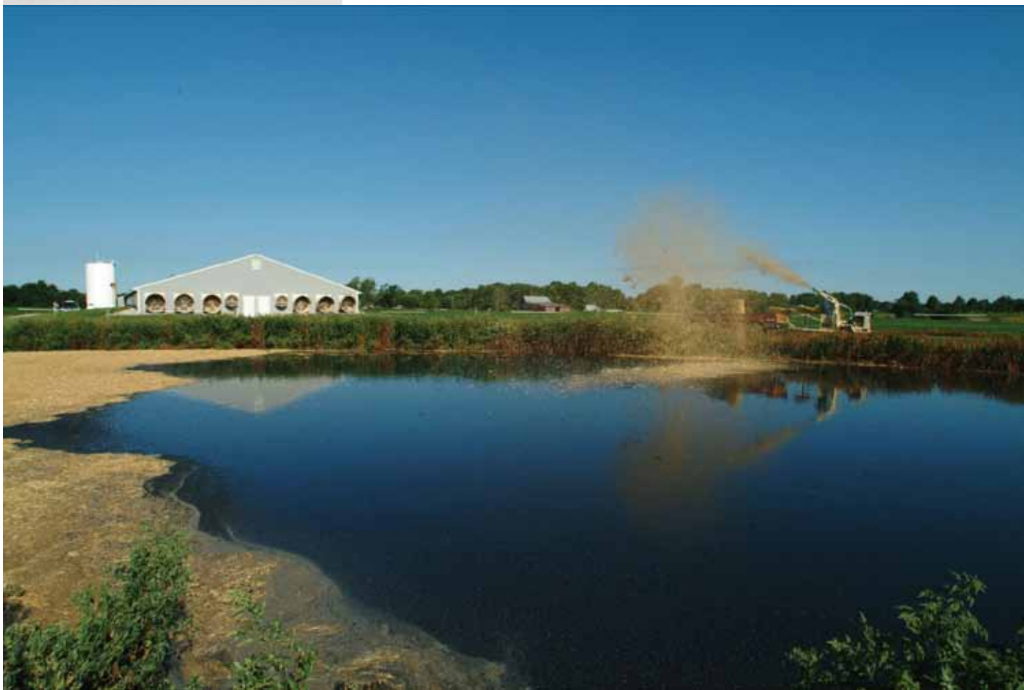
Figure 2. A straw cover being installed on a manure storage structure. Straw must be replenished frequently to maintain cover effectiveness. (Photo courtesy of the Pork Checkoff)
