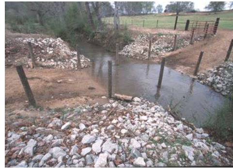
Figure 3. Fenced stream crossings allow animals to get to pasture on both sides of the stream. Concrete or stone on the stream banks helps control erosion.
